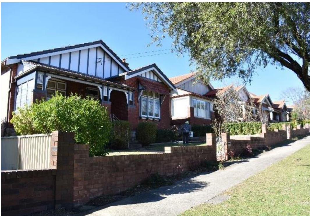
Image 7: Contributory dwellings in the study area. The consistent roof lines of several dwellings can be seen here. Source: Bayside Heritage Study - Review of Heritage Conservation Areas (2019)
