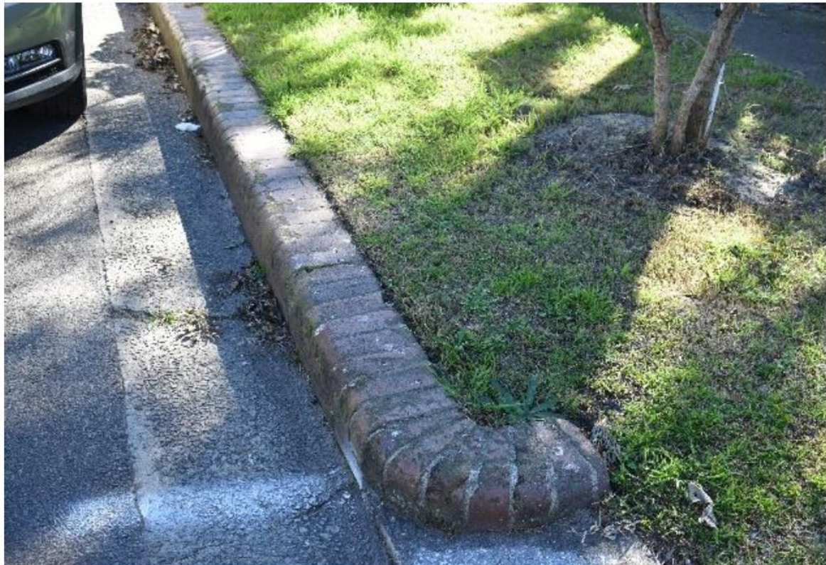
Image 13: Brick kerbing- an example of a historic streetscape element. Source: Bayside Heritage Study - Review of Heritage Conservation Areas (2019)
