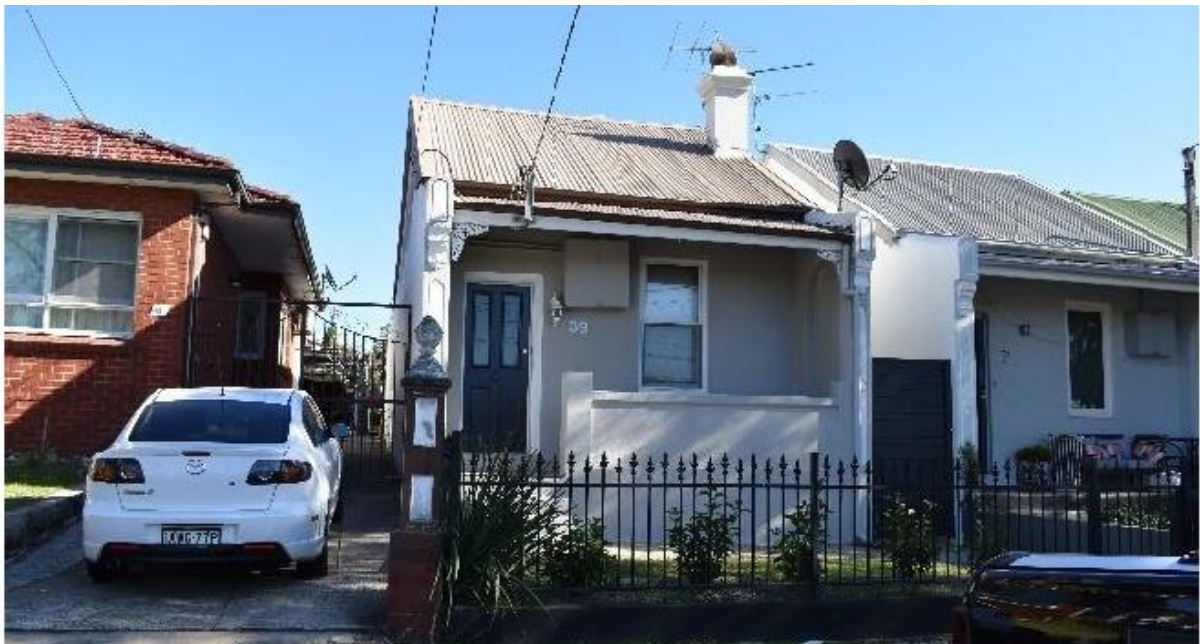
Image 1: An example of a Jackson's Row cottage. Source: Bayside Heritage Study - Review of Heritage Conservation Areas (2019)
